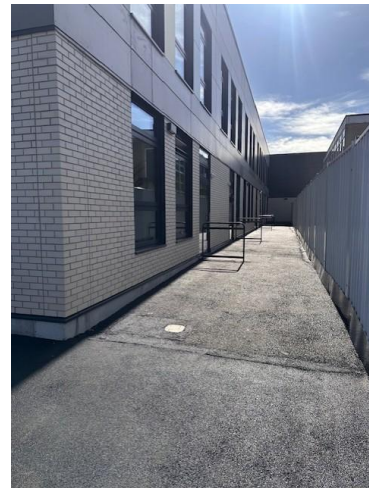
KS1 classroom doors in the new building
